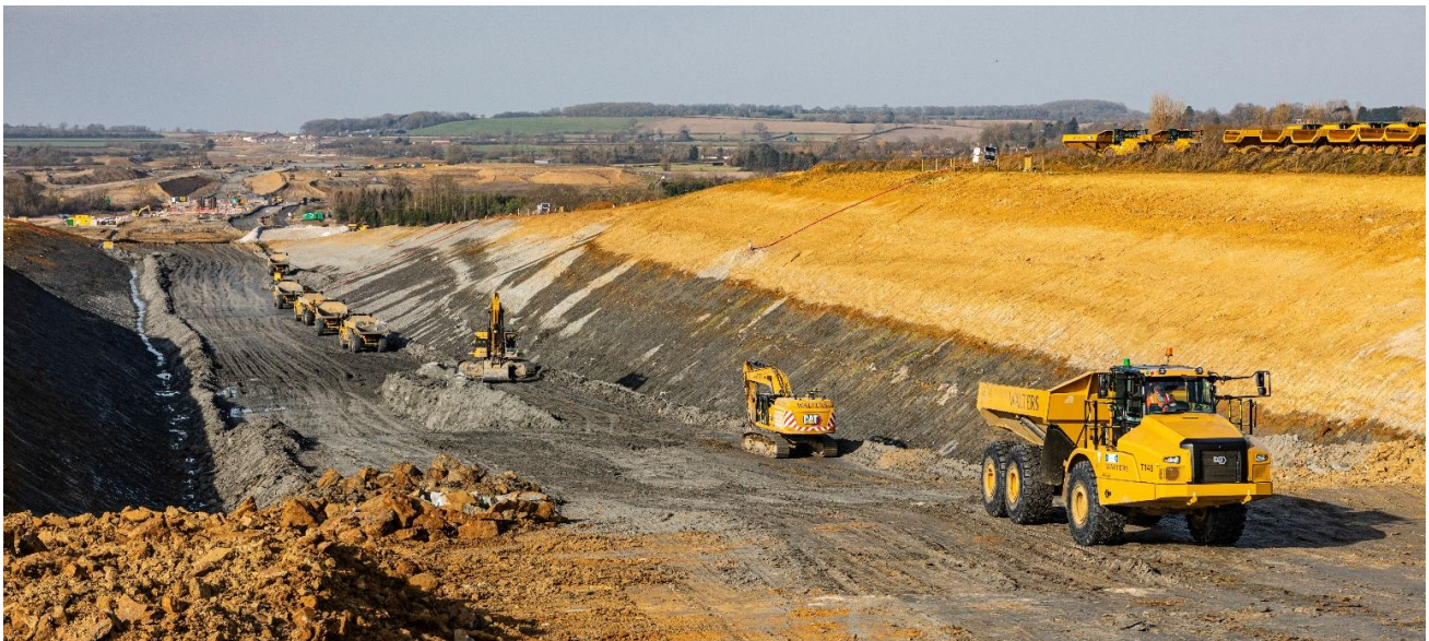
HS2 Railway Cutting in Construction
